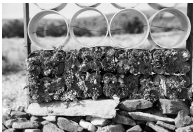
Figure 18. Vertical green wall with closable blind made from recycled pipe.
